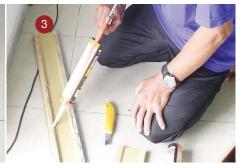
Put the power nail glue and install the skirting cornice.
