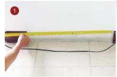
Put the end skirting-cornice on the end of wall. Measure the length space between the end skirting-cornice with skirting cornice as shown as picture.
