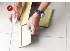
Cut off the cornice length that we get from the 1st method. Use hot glue to stick the end skirting-cornice with skirting cornice as shown as picture.
