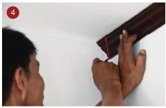
Mark line from the cutting point to corner of the wall as shown as picture.
