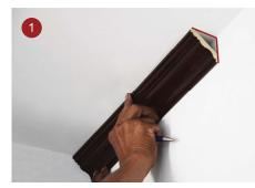
Place the cornice to fit the corner of the wall and ceiling.
