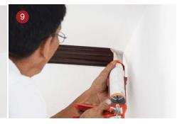
Put the power nail glue on the connecting point as shown as picture before installing the next cornice.
