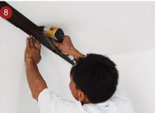
Put the power nail gun instead of supporting the cornice on 3-5 minutes.
